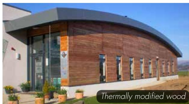
A thermally modified timber developed during collaborative research with local companies has been used to clad Halen Mon’s new Saltcote building on Anglesey. Larch timber from Welsh forests was thermally treated at the UK’s only active thermal modification kiln on Anglesey for the elegant new building.
